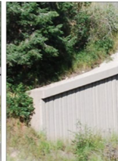
*D | Turning the ends of walls helps integrate them into adjoining slopes.*
