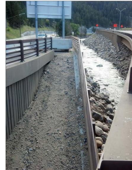
*C | Underpasses that utilize open-span bridges offer greater visibility for wildlife than box culverts or enclosed crossings.*
