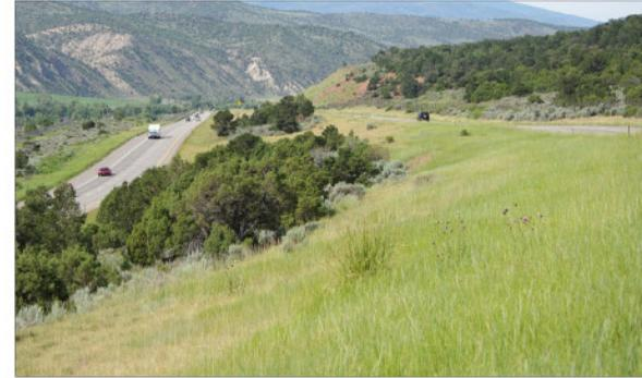
A | Rounding the top and toe of the slope blends embankments into the existing landscape and facilitates
