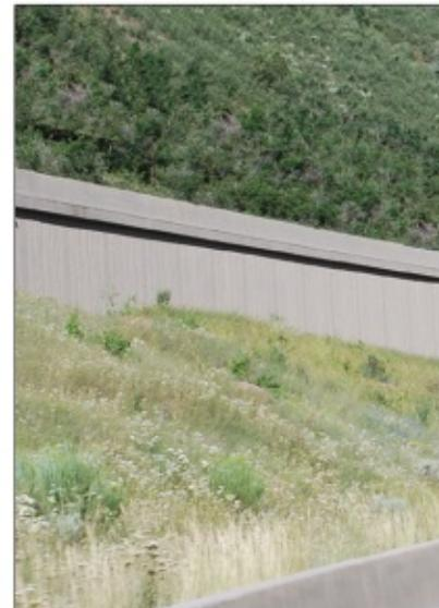
*C | Incorporate earthwork solutions in conjunction with structured retaining to limit the height of retaining walls.*
