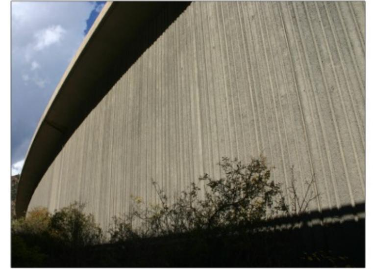
*B | Simple vertical textures provide depth and shadow to large wall faces.*
