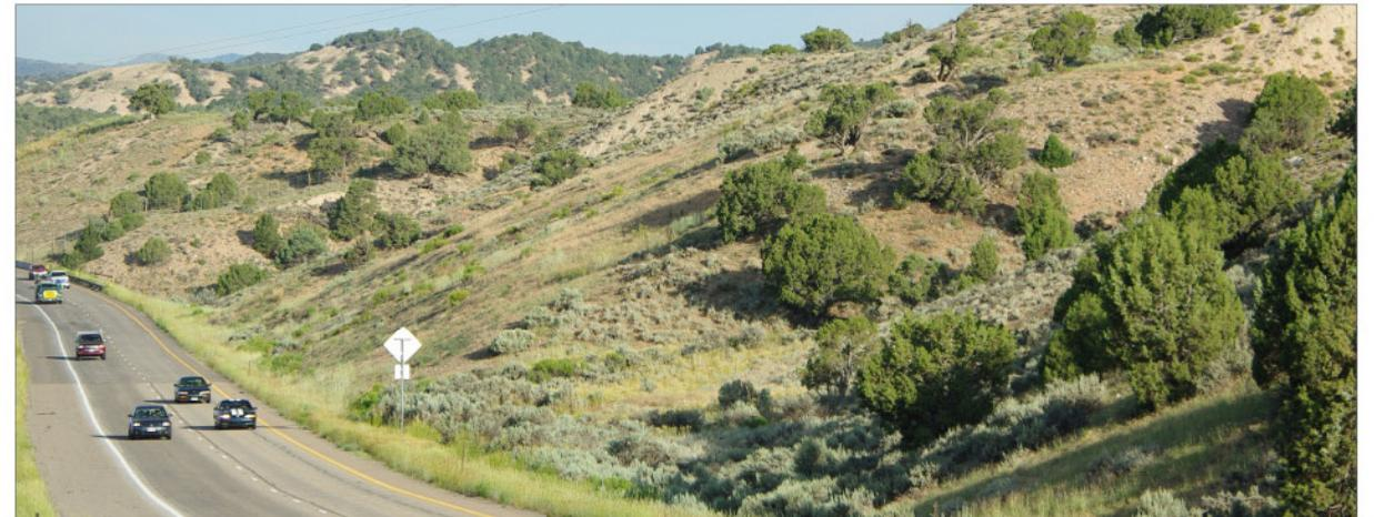
D | Utilizing variable slopes through the length of an embankment mimics the natural patterns found in the
