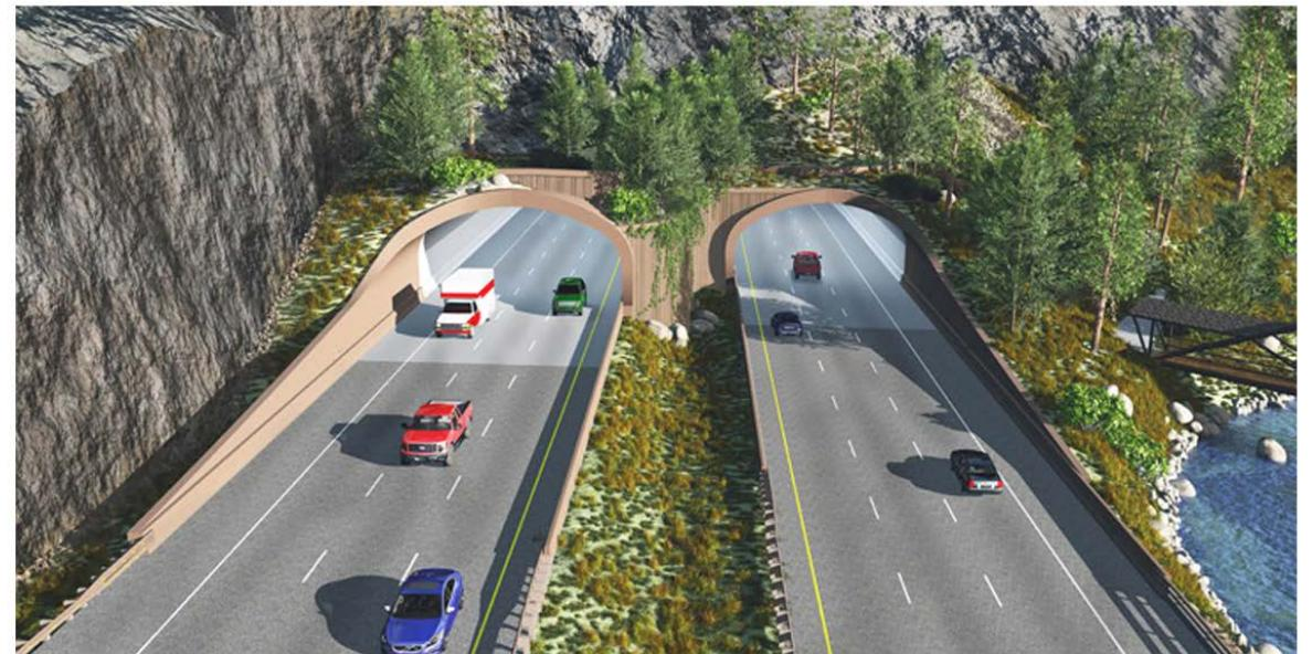
C/ The transportation facility at the Twin Tunnels aids in rock fall protection by incorporating rock fall protection into the design of retaining wall, noise wall, grading and landscape.
